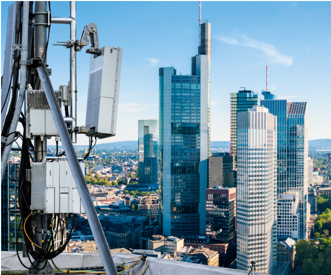
Example of mMIMO Active Antenna System
