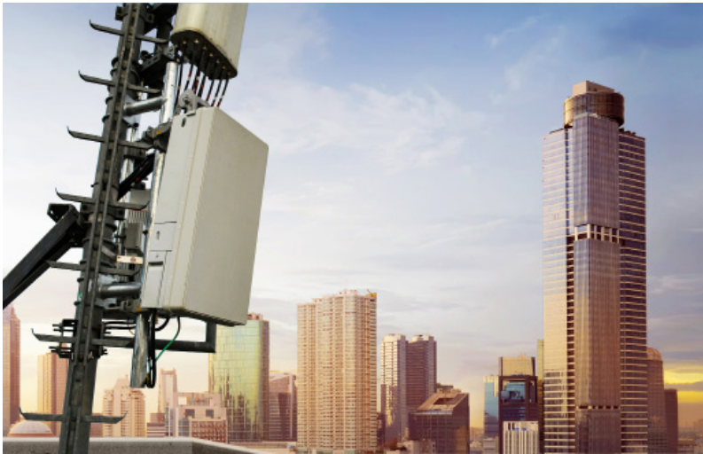
Example of mMIMO Active Antenna System
