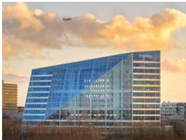
The Edge Building, Amsterdam photo © Ronald Tilleman
