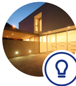
Lighting Management Systems
